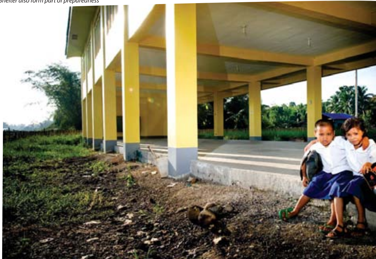
Shelter also form part of preparedness
