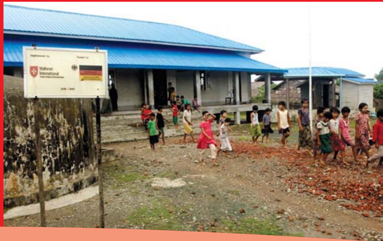
A school cyclone shelter.
